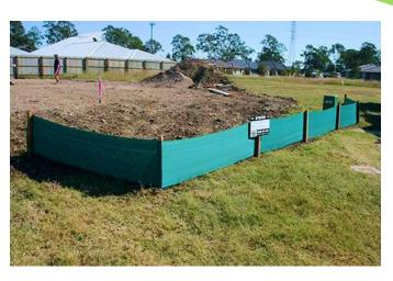
SpillSmart Silt Fence has been designed to assist with erosion control and the prevention of sediment and soil runoff from earthworks, construction sites and roadworks. Suitable for both civil and domestic projects, a silt fence allows water to freely pass through whilst preventing sediment and other matter from reaching stormwater inlets, waterways or travelling across worksite boundaries.
